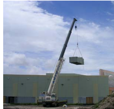
F26. RTU Removal for future re-installment
