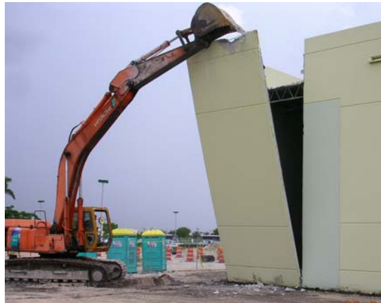
F20. First Panel Removed on West Wall.
