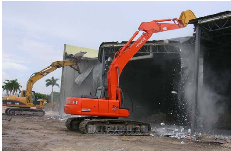
F21. Roof System Removal after Columns & Joists Were Burned
